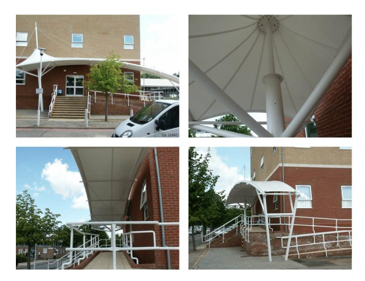
J & J. Carter Ltd were commissioned by the client to design and build a new canopy to the original scheme as designed by Sutton Griffiths. The new canopy has been built using a welded steel frame work, with stainless steel tension cables and a White PVDF lacquered PVC fabric.
