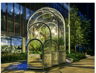
J & J Carter were contracted by Cake Industries to manufacture and install the membrane roof for an arched greenhouse, named the Hothouse. Designed by Studio Weave the structure is built from a series of galvanised steel arches and steel tension cables with a transparent membrane, as part of London Design Festival.
