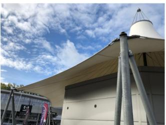
J & J Carter were contracted to design and build a tensile fabric canopy to cover the outdoor sales area. The canopy had to interface with an existing building, which could not resist the canopy loads.
