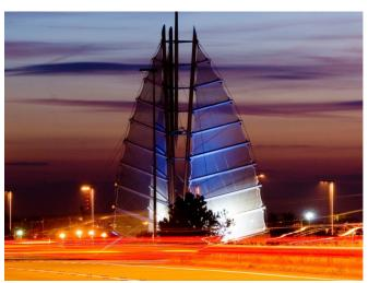
J & J Carter was appointed to manufacture and install the fabric for the 43 metre tall tri-sail structure that is the landmark to the entrance of the city.
